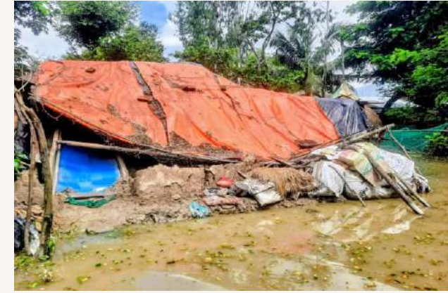
Collapsed shelters reflect the urgent need for humanitarian intervention.
